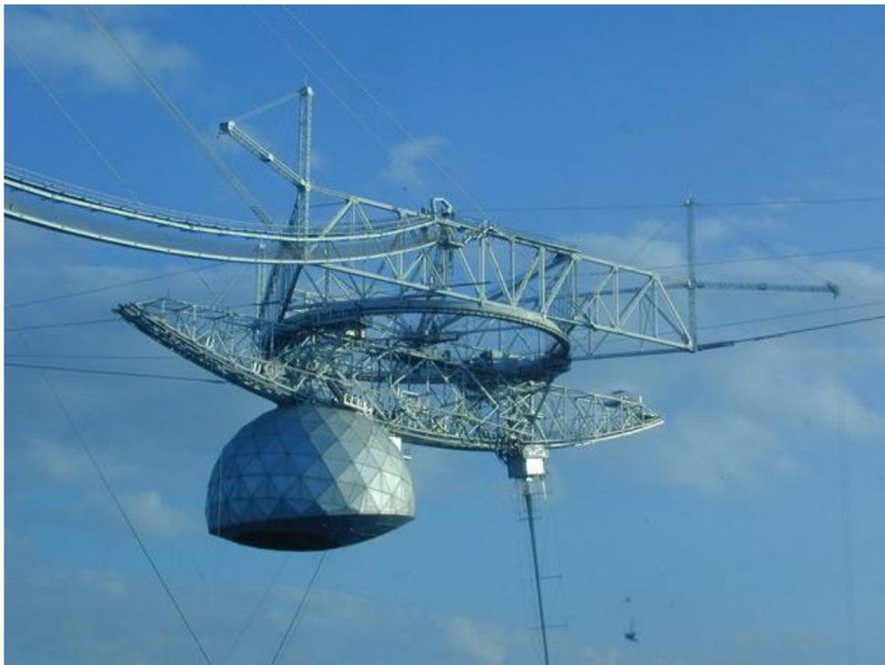
*The 430 MHz radar line feed is seen extending to the lower right in this image. Credit: USRA*
